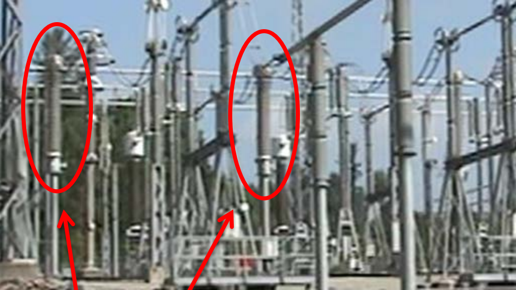
CVTs or PT under test
