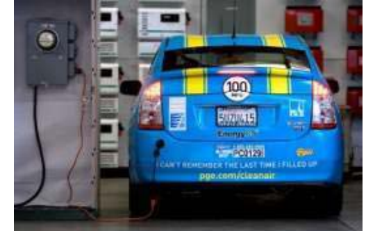
Smart charging for electric vehicles
